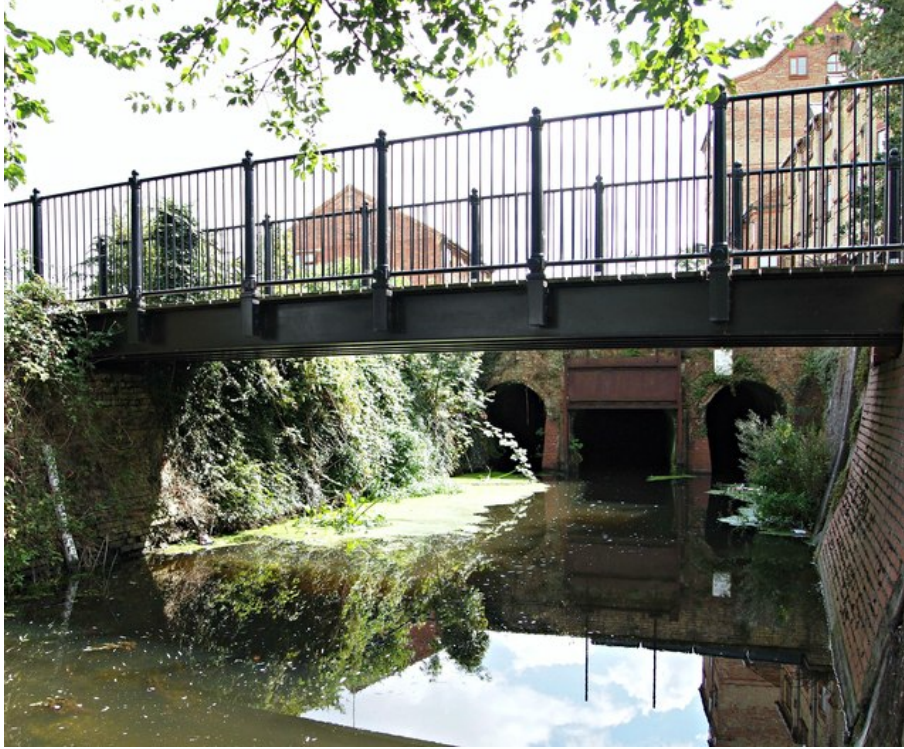
Figure 1.1: A typical steel beam footbridge.[3]
