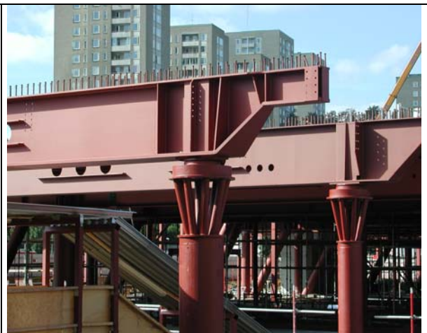
Detail of steel support structure
